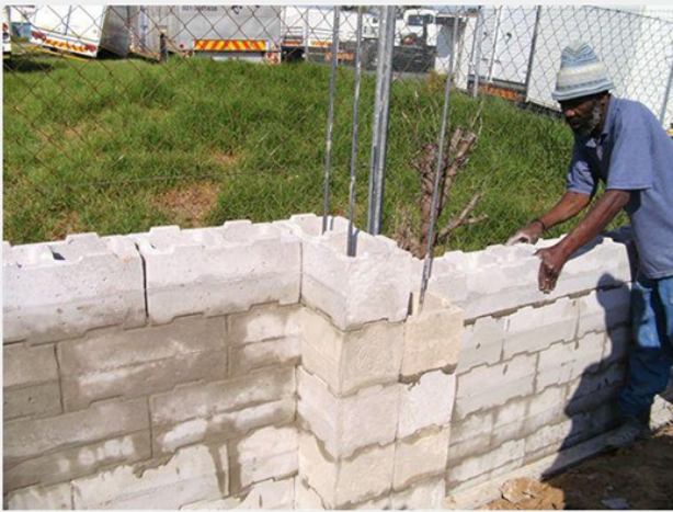
Example of control joint ↑ cut afterwards with a grinder.
