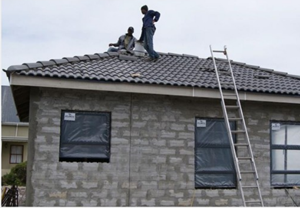
Example of control joint ↑ cut afterwards with a grinder.
